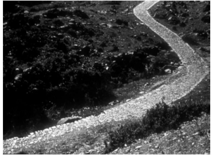
Roman Road going left and right
